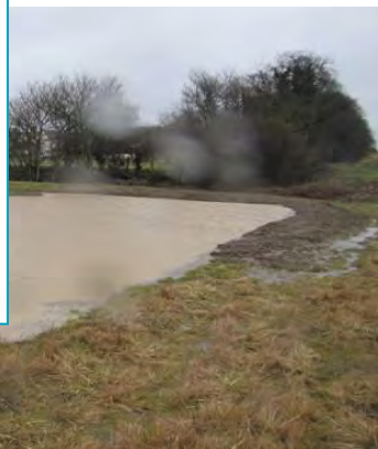
Bunding on low slopes for impermeable soils
